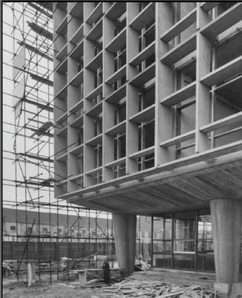
assemblage of schokbeton facade panels
