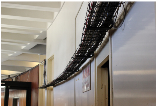
Figure 21. Detail view of data trays.
