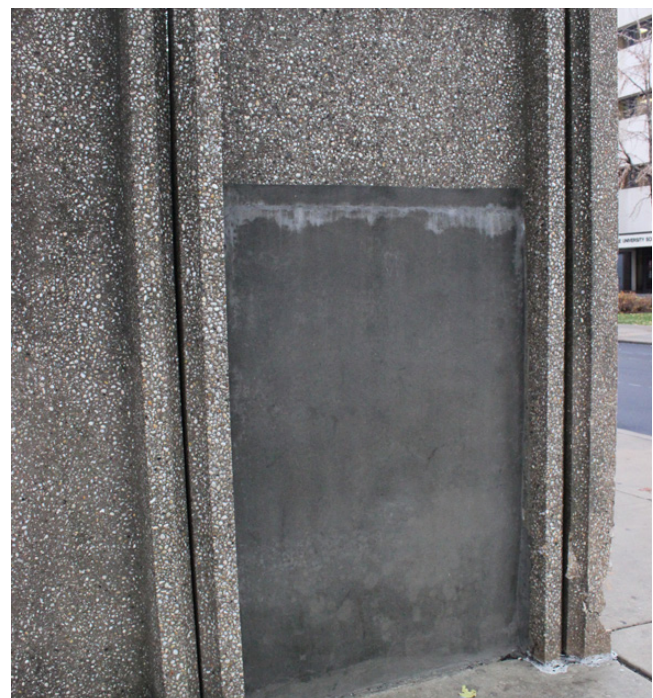
Figure 31. Detail of inappropriate concrete infill.
